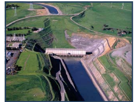
Banks Pumping Plant
