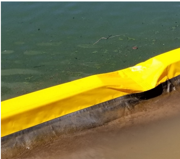
Turbidity curtain showing effectiveness
