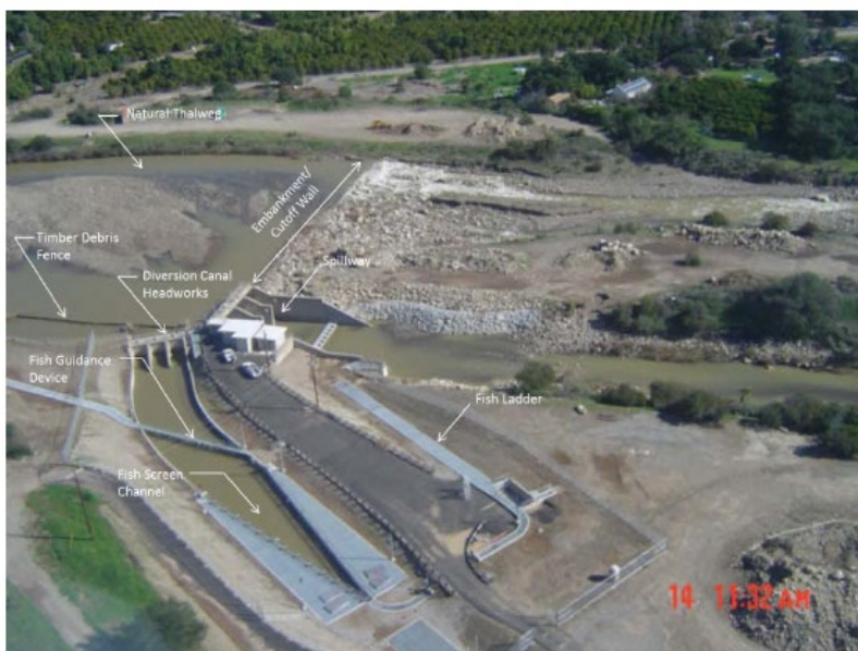
Figure 5-5. Robles Diversion Fish Screen (MKN Associates, 2019)
