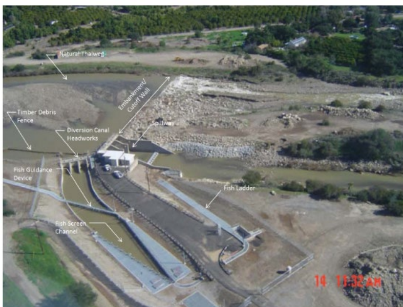
Figure 4-5. Robles Diversion Fish Screen (MKN Associates, 2019)
