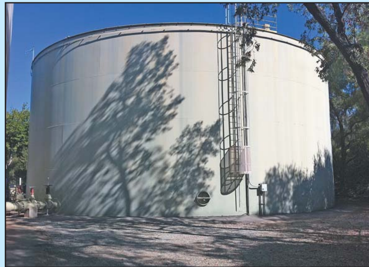
Casitas' Ojai 4 (M) Reservoir Tank.
