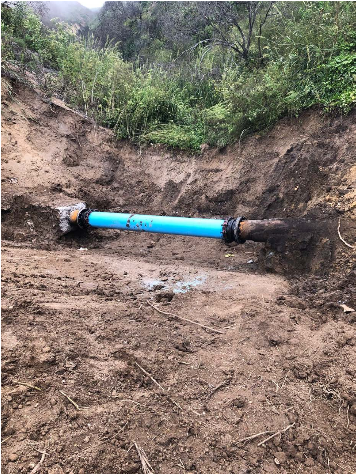
Finished Repair from June 2019
