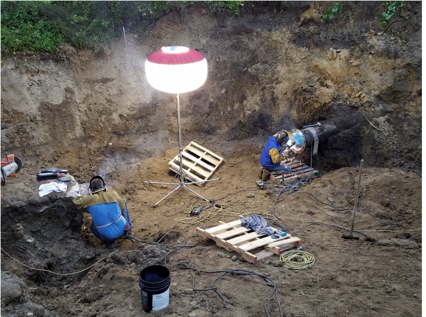
Repair Work from June 2019 Mainline Break
