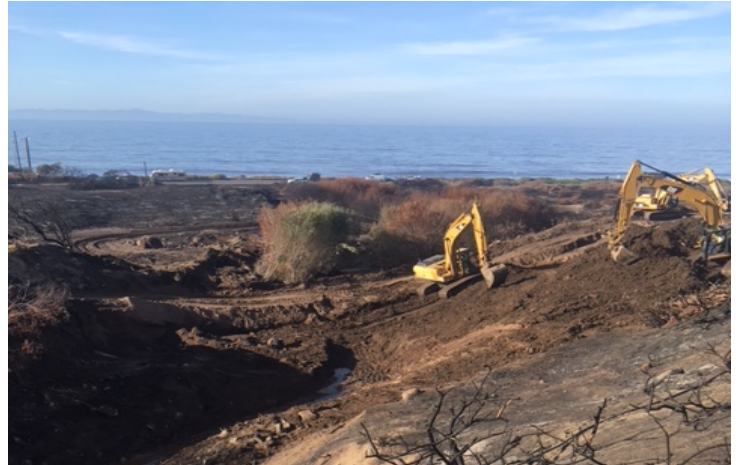
Burying the New 10" Replacement Line
