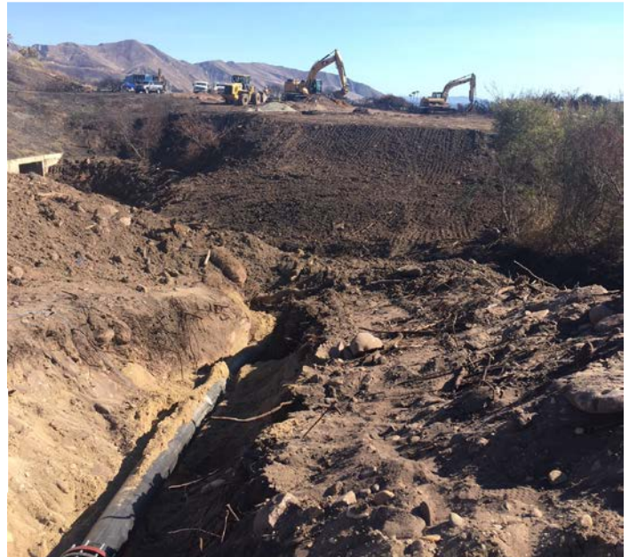
Construction Nearing Completion (10" Replacement Line in the Foreground)
