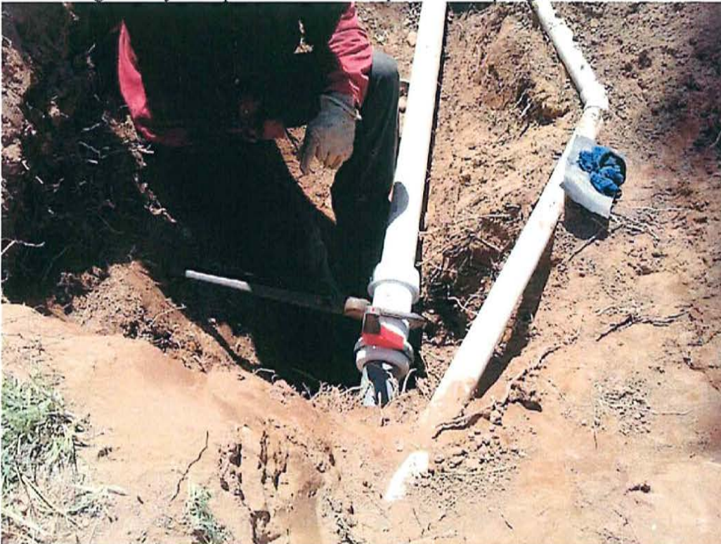
Line in neighbor's yard repaired with 3" compression coupling.
